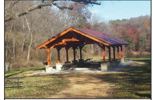
Newly constructed shelter at Stewart Lake County Park in Mt. Horeb
