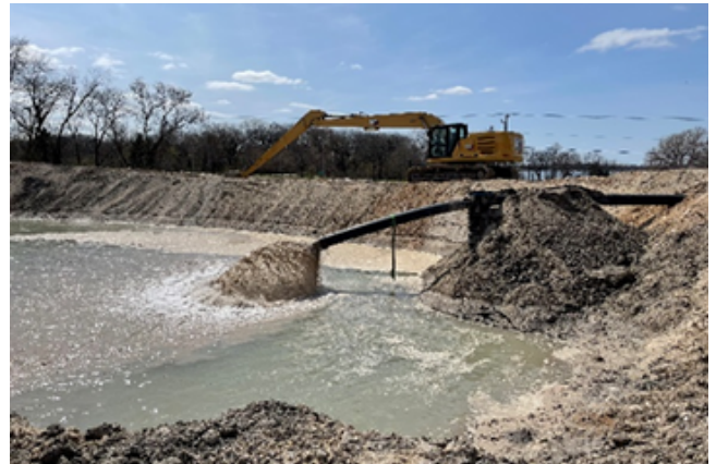
Dredge equipment removes sediment and water from riverbed (left) and pumps it to a dewatering basin (right) where the sediment settles out before the water is returned to the stream.
