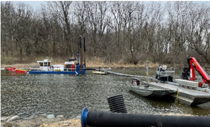
Dredge equipment removes sediment and water from riverbed (left) and pumps it to a dewatering basin (right) where the sediment settles out before the water is returned to the stream.
